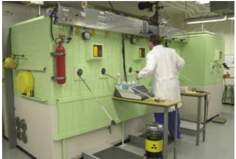
The front panels of RotoPol-15 and RotoForce-1 (above, over the cell) are placed outside the hot cell together with the Multidoser dosing unit (on the table)
